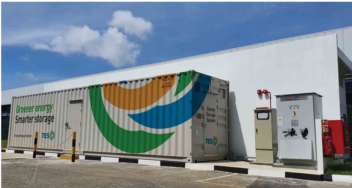
TES B facility equipped with second life containerised battery energy storage system
